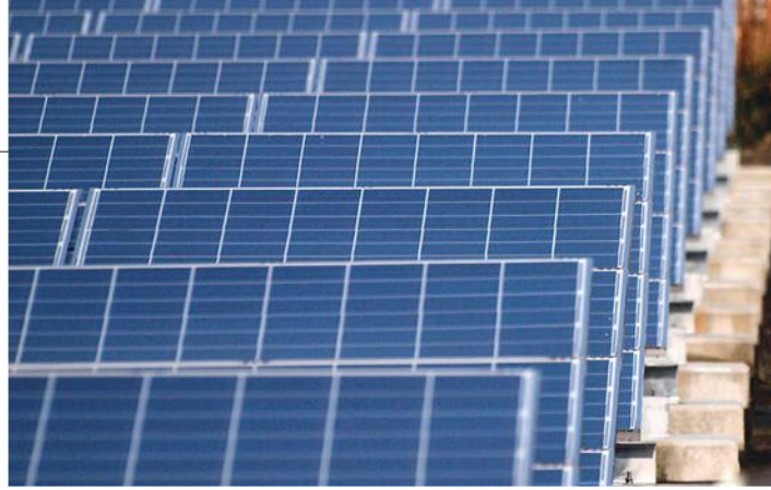
SunPower's prototype solar panel converts 24.1% of the sunlight that hits it into electricity, making it vastly more efficient than conventional solar cells, which are usually between 15% and 18% efficient. (Image courtesy of coniferconifer, Flickr)
